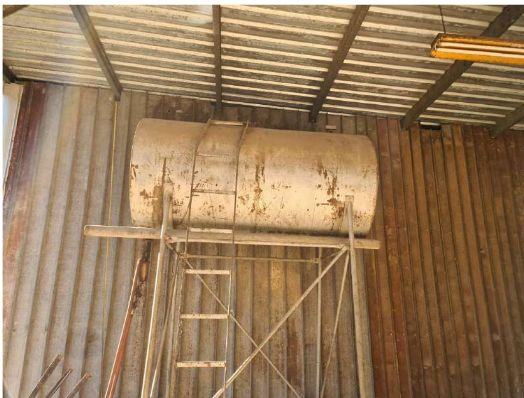
Photograph 13: AST tank with apparent fuel dispenser.
